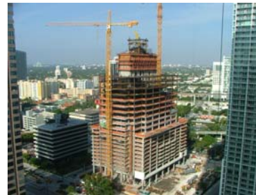
Brickell Financial Center Client: Southern Steel Tons: 4020
